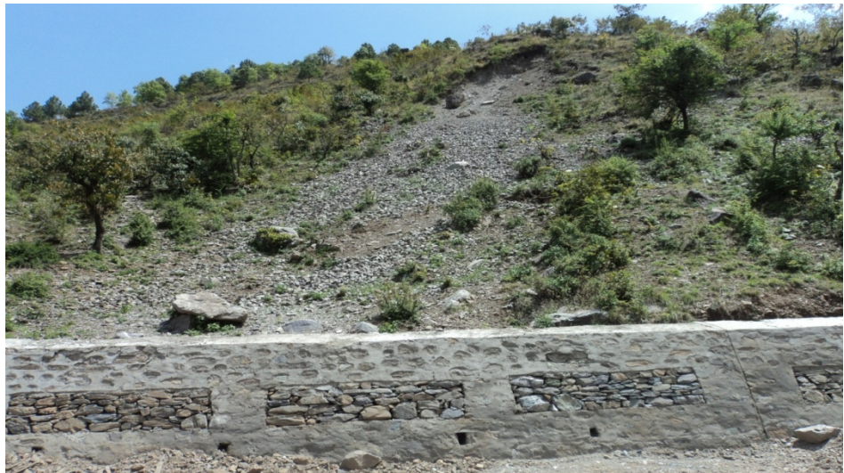
Photograph 1: Mitigation Measure – Breast wall on the road of Contract Package-17
