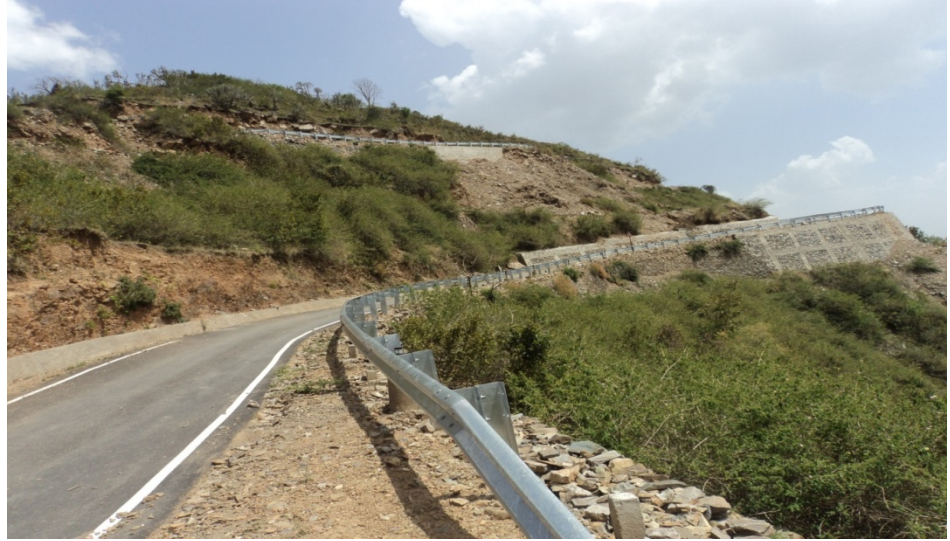
Photograph 2 : Mitigation Measure – Gabion with Wirecrete on the road of Contract Package-17
