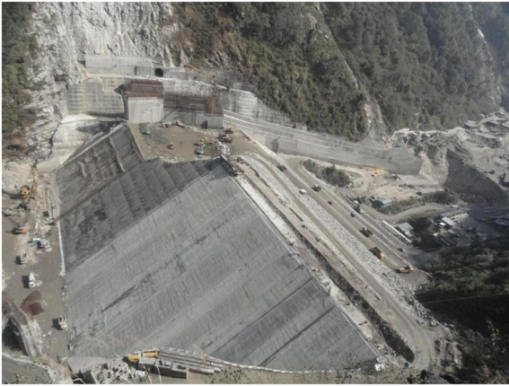
Photo 1 Teesta-III CFRD in final phase of construction (2013)
