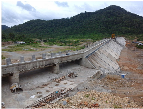
Photo 2 Stung Tasal CFRD before reservoir filling (March 2014)
