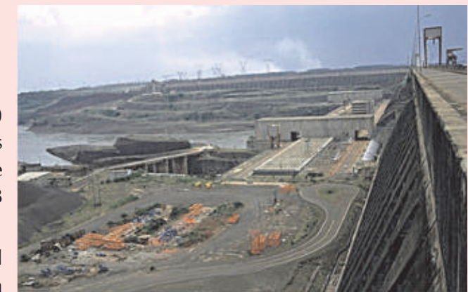
On top of the 7.6 km dam, a 12 800 000 m 3 of concrete was used for the project ITAIPU.
