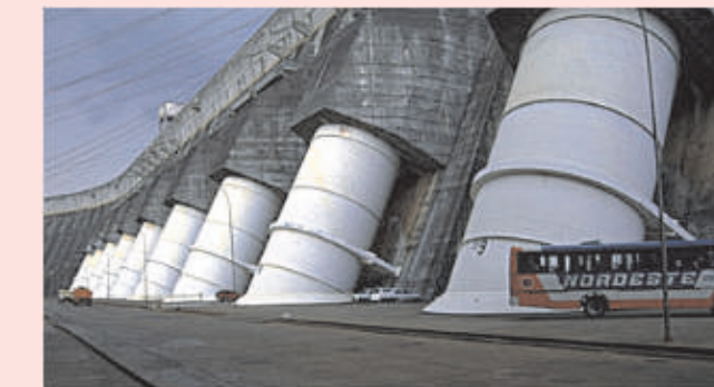
Total view of the ITAIPU power plant Left part shows overflow (spillway), the power station is located in the middle
