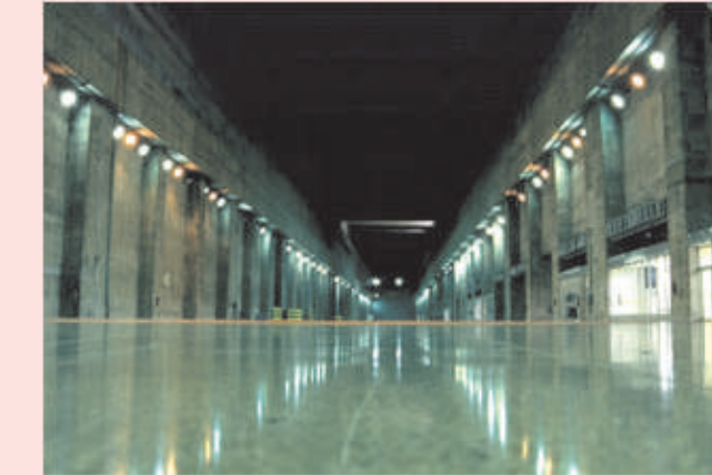
Inside the ITAIPU Powerhouse Dimensions: Length 986 m, Maximum height 112 m and width 99m. The red line on the floor indicates the border of Brazil and Paraguay.
